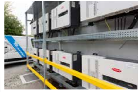
Ausbau Photovoltaikanlage Expansion of photovoltaic system
